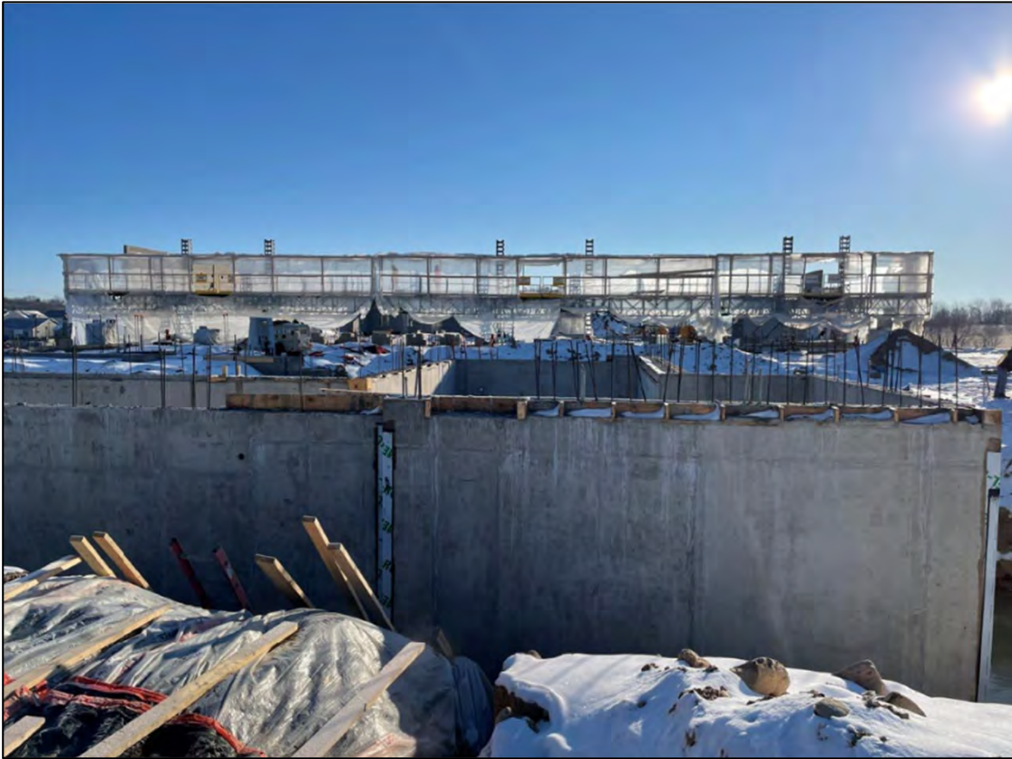
Basement Foundation Walls (foreground) Masonry HydroMobile setup (background is PD)
