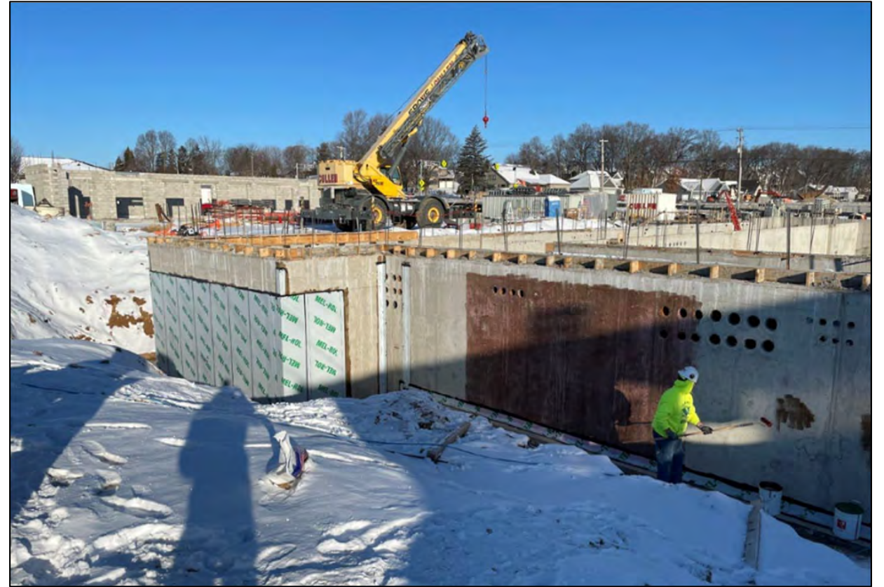
Basement Foundation Walls (foreground) Masonry Walls at FD (background)
