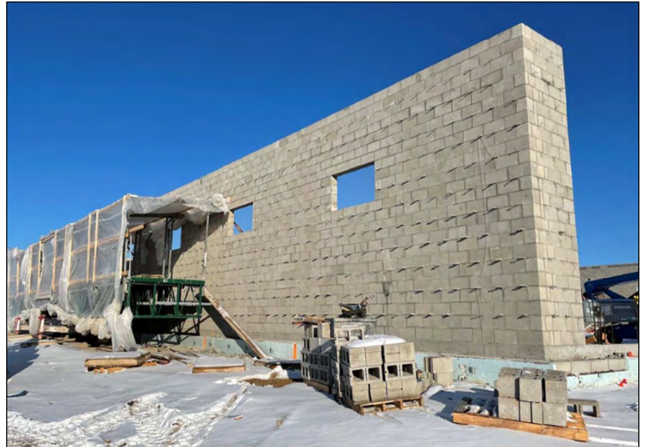
Masonry at Police Garage
