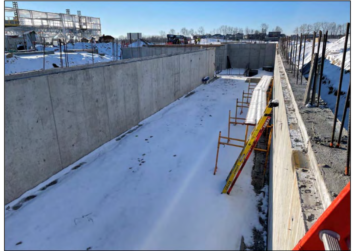
Foundation work at Basement and Elevator
