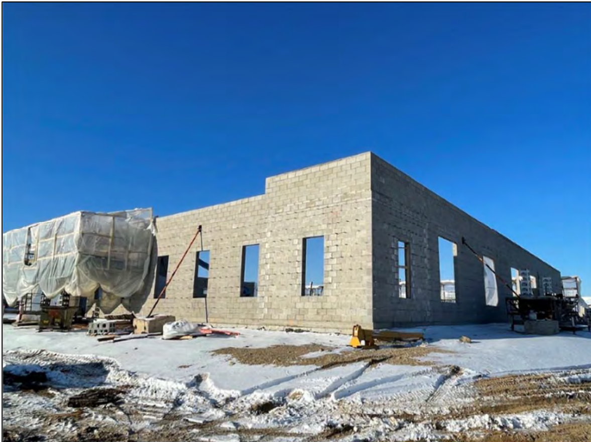
Masonry at Police Unit
